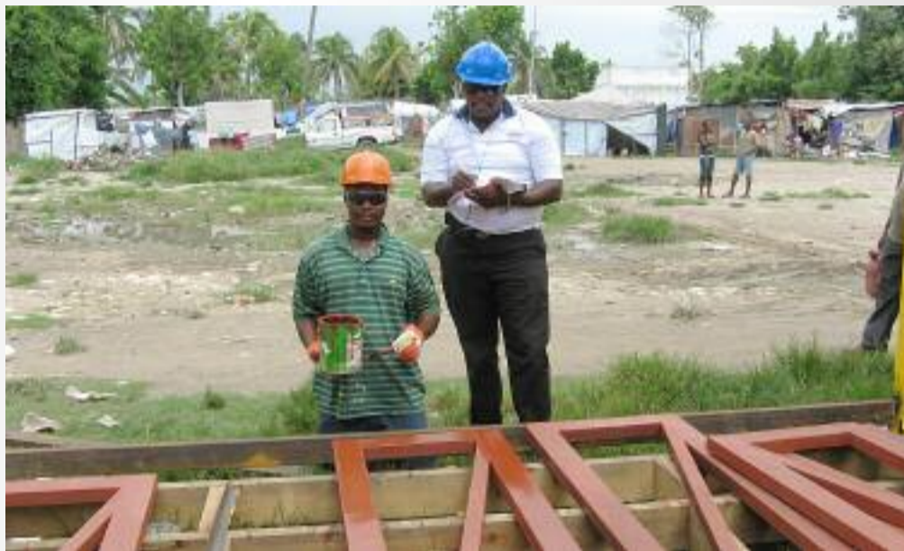
Applying primer to prefabricated beams under supervision of project staff
